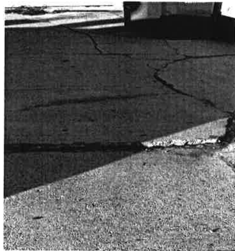
Driveway lifted by Roots of Tree
