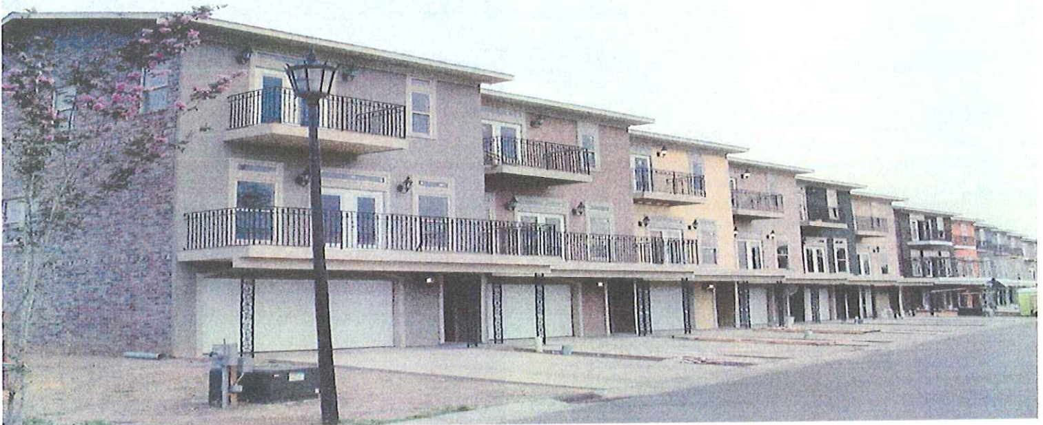
FRONT SIDE VIEW OF RESIDENCE. PICTURE TAKEN 10/25/07.
