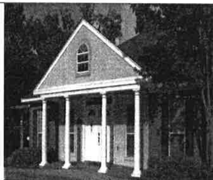
Our Front Door-Left Porch on building
