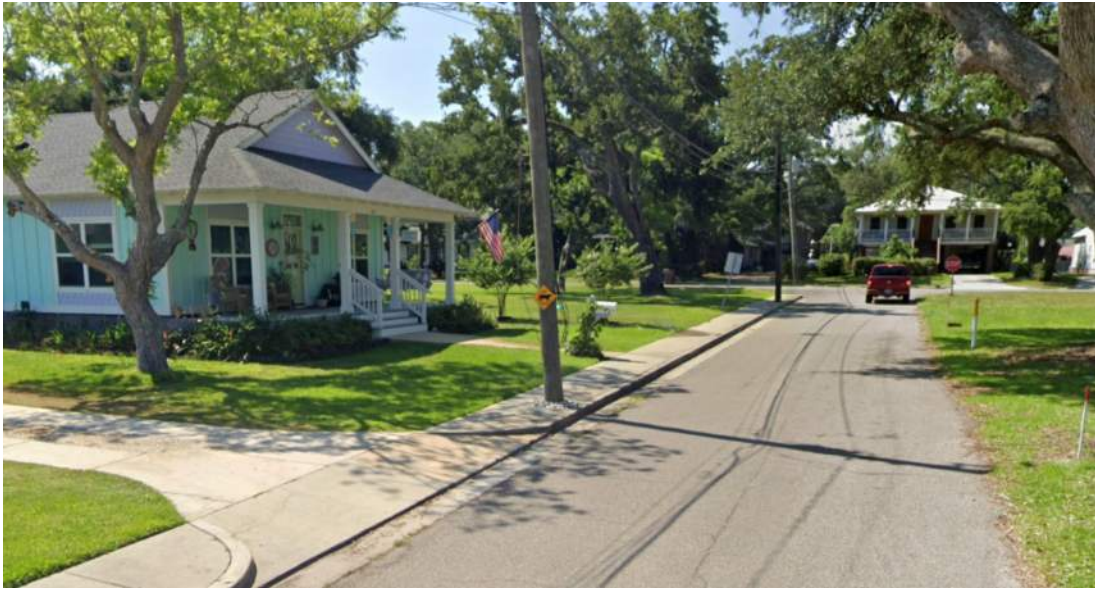
Figure 1: Obstruction Within Pedestrian Access Route
