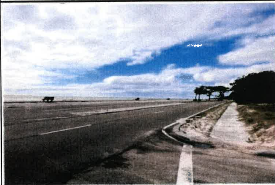
View looking west down Beach Blvd (Hwy 90)
