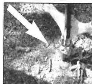
Figure 17. Reducing soil compaction using high-pressure air injector. Cracking of soil indicates some relief from compaction.
