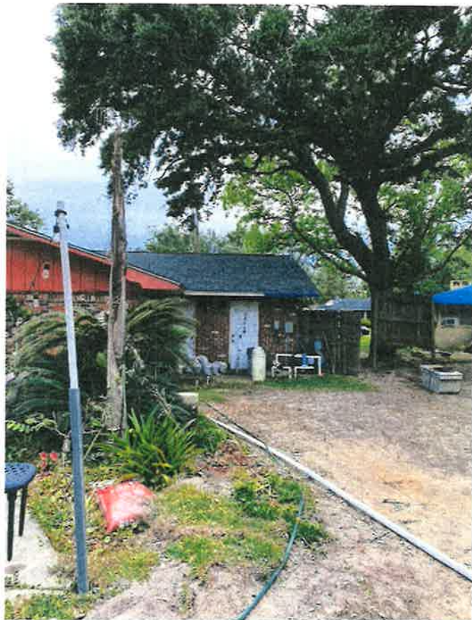
Tree Roots & tree hangs over house
