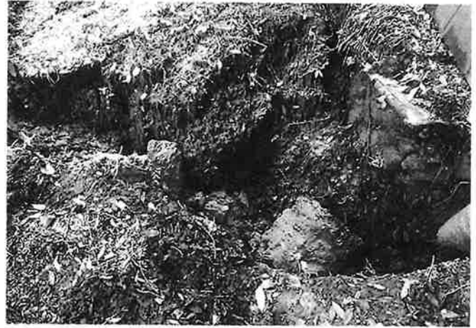
1010 Pino St. - Drainage Sinkhole
