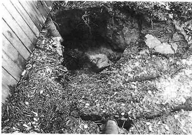
1010 Pino St. - Drainage Sinkhole
